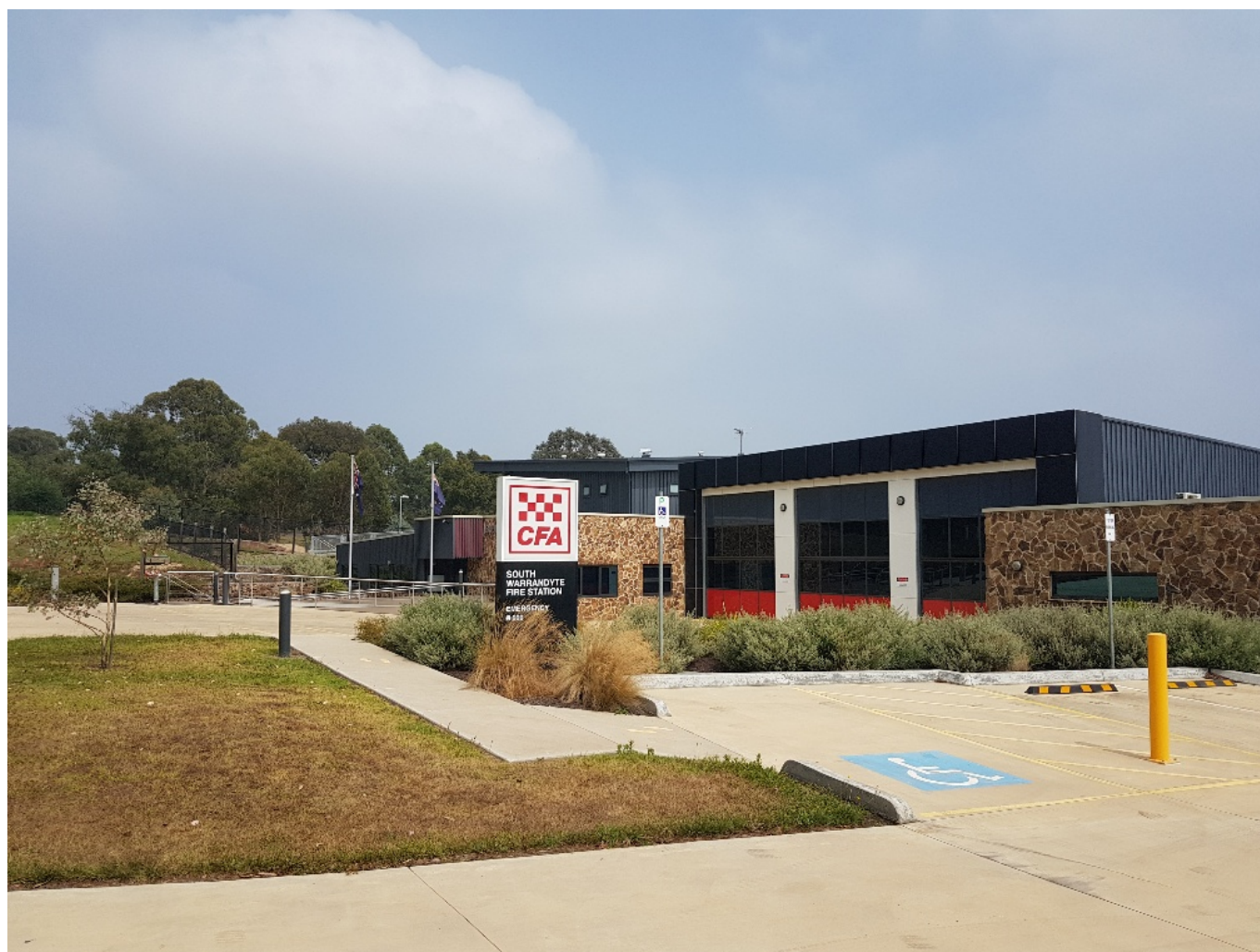
A CFA fire station on the outskirts of Melbourne.
