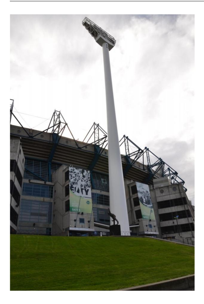
The diameter of each hollow steel tower at the base is 4 metres, narrowing to 2 metres diameter at the top. On top of each tower is around 140 lamps. I must say that, when the MCG lights are turned on, it's like it is day time again. The ground and all the stands are so bright and vivid. It makes you happy and excited just to be there.
